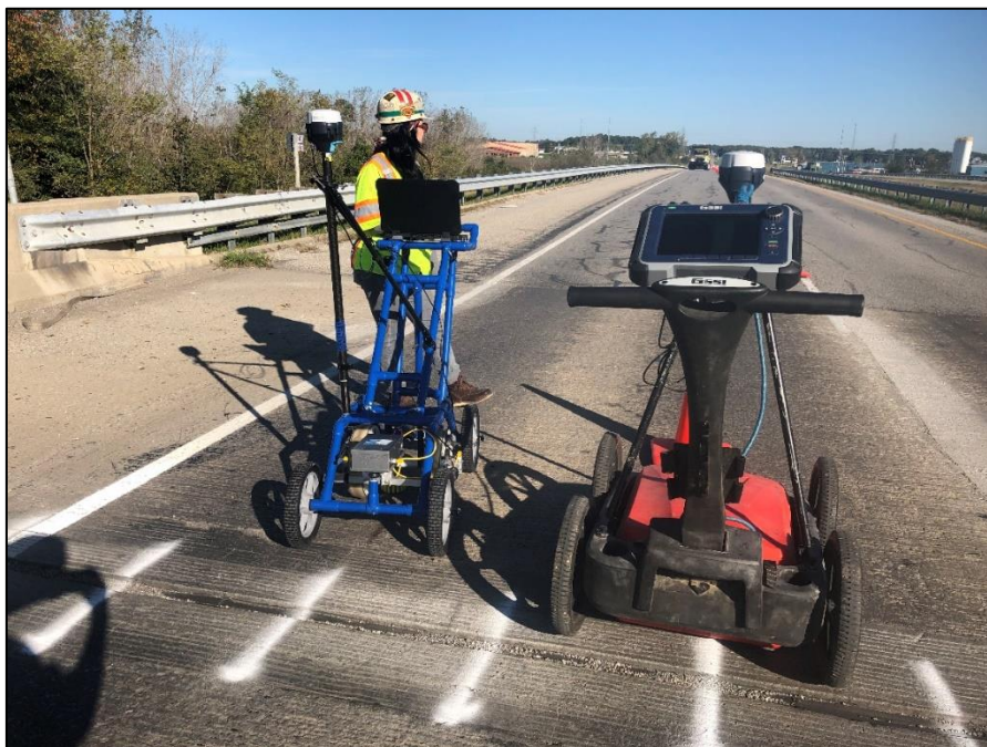
Figure 14: Photograph of Olson Sonic Surface Scanner – Impact Echo system (left) and of the GSSI SIR-4000 computer and a 1600 MHz GPR antenna (right) placed in a hand push-cart for ground coupling. Note GPS unit antennas (white) sticking up above each cart
