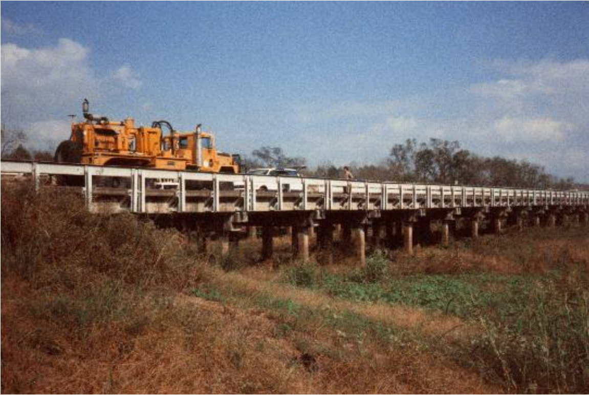
Figure 6: Vibroseis over Pile Bent on Trinity River Relief Bridge No. 4
