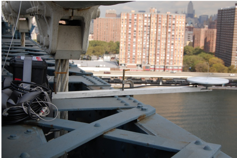
Figure 4. GPS receiver mounted on Manhattan Bridge
