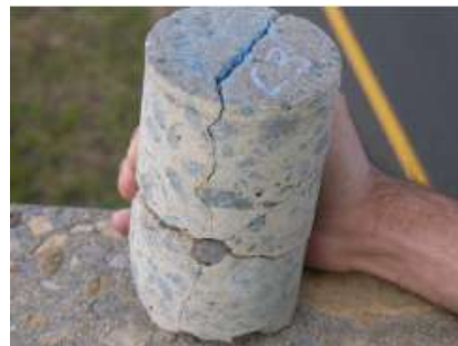
Core # 3 - Delamination Depth at 3.5 inches
