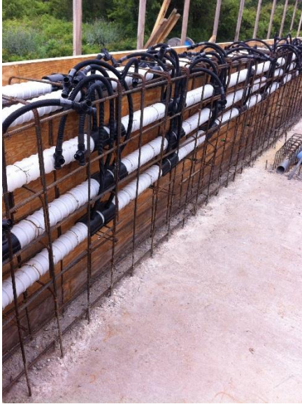
(a) Corrugated plastic ducts within the web and flange of the South Wall
