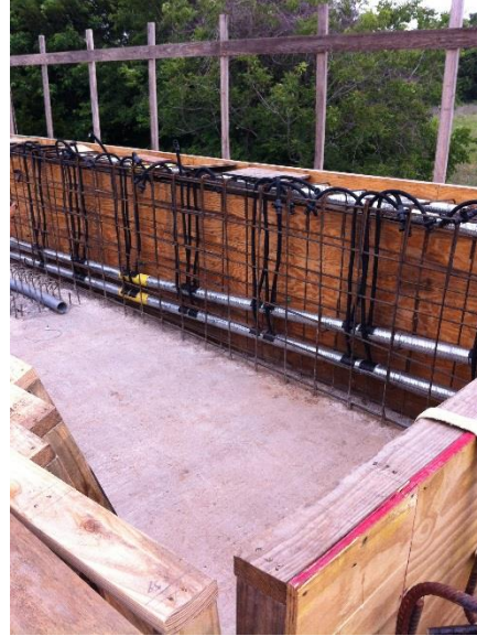
(b) Metal ducts within the web and flange of the North Wall
