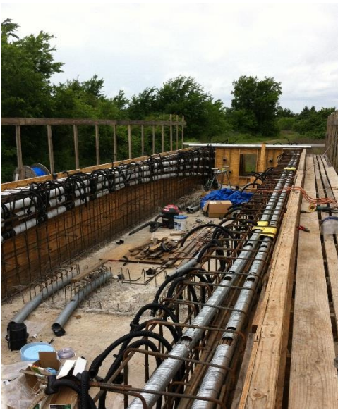
(c) Draped internal tendons
